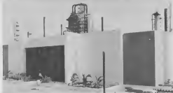
The newly expanded Refining Control Center.
